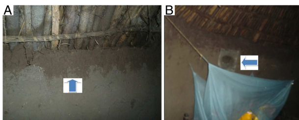
Figure 3 Openings around eaves closed by mud (A) and openings for ventilation closed by metal mesh (B).
